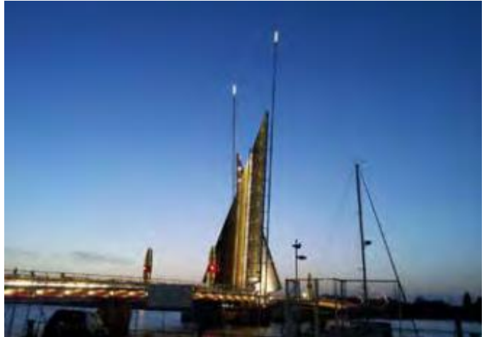
Twin Sails Bridge – Source: BCP Council
