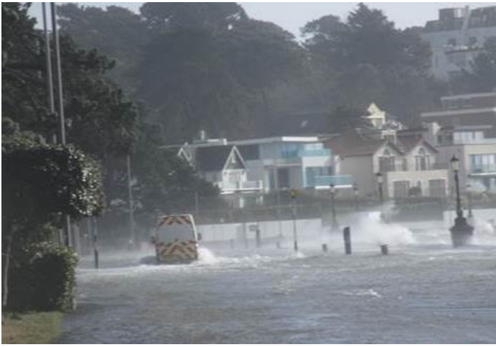
Breaching of the Sea Wall at Shore Road (February 2022) – Source: Steve Malpass
