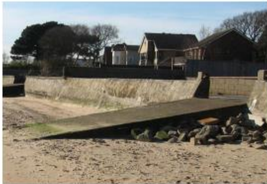
Figure 10: this slipway has been constructed as a solid mass of concrete which results in a complete loss of natural, intertidal habitat under the concrete and the total displacement of tidal water. There has been no mitigation for the structure's adverse effects such as meshing, open piling, or seasonal removal.
