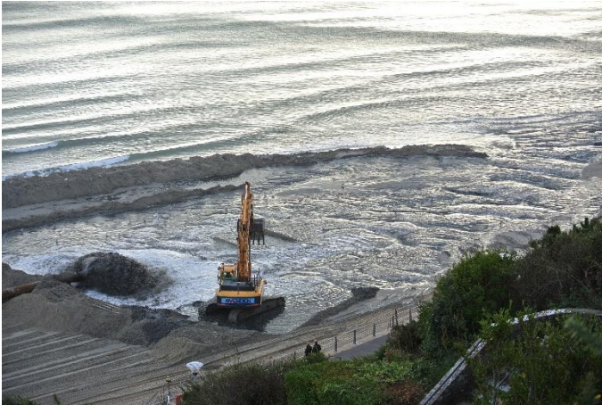
Poole Beach Replenishment – Source: PHC
