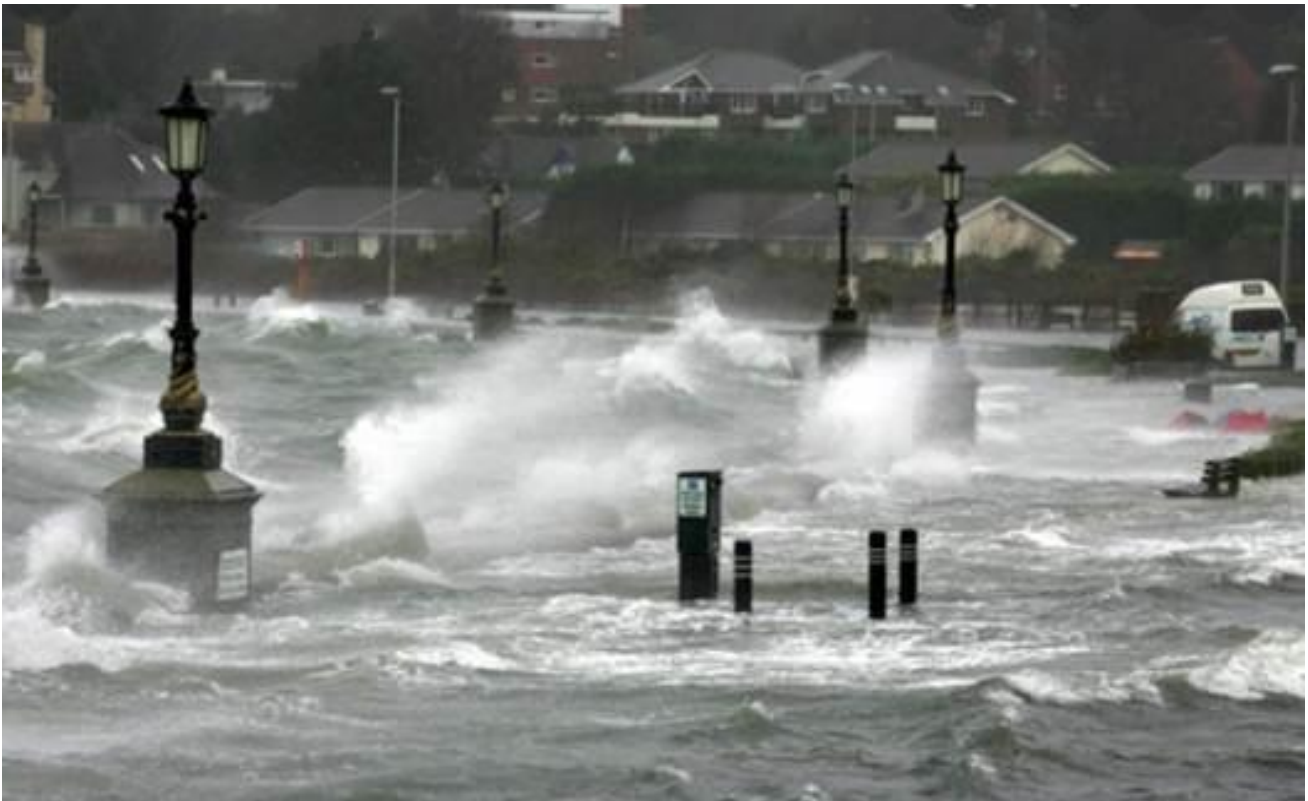
Coastal Flooding at Shore Road (February 2022) – Source: Steve Malpass
