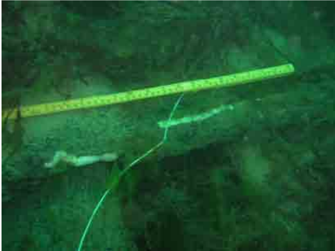
Figure 3 Shipworm tunnel 500mm long on shipwreck timbers
