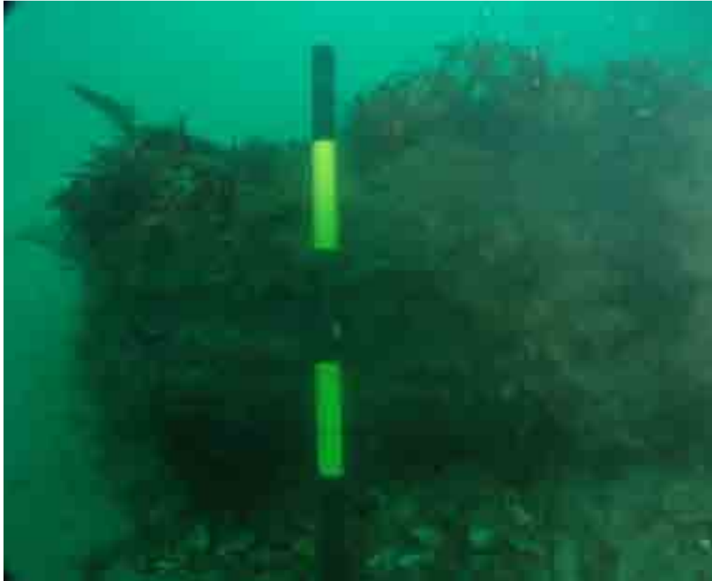
Figure 14 Showing undercutting at foot of feature as seen 13 th November 2006
