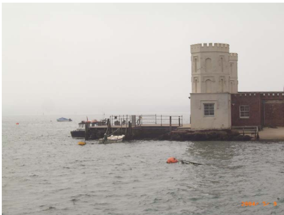
Photograph 17.3 Engineered shoreline around Brownsea Castle
