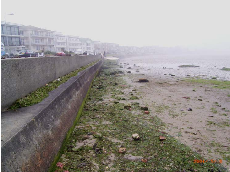
Photograph 17.1 Seawall adjacent to Shore Road in the Whitley Lake area
